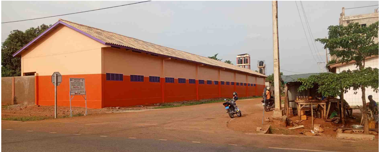
Back side – exterior paintwork complete
